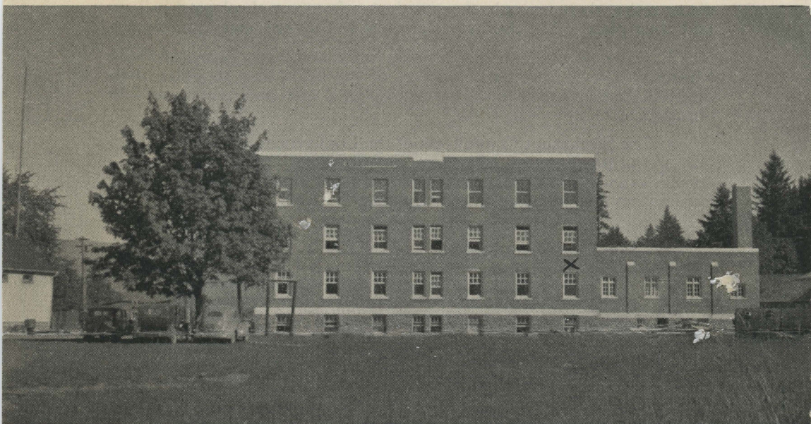
Alberni Indian Residential School, to be opened this fall
