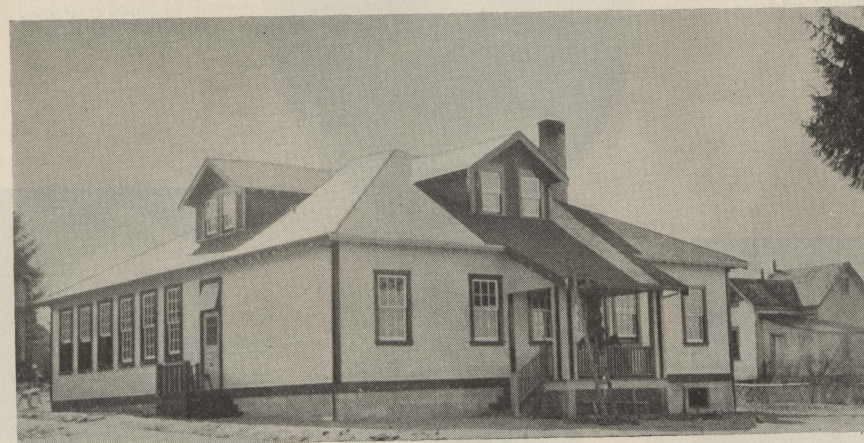
Day School and Teachers' Residence, Port Simpson, erected 1938
