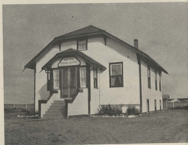
Below: Mitchell Memorial Hospital, Carrot River, Sask., erected 1935
